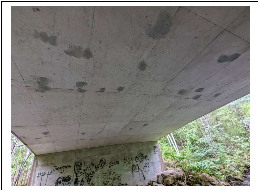
Photo 10 Typical deck soffit with previous concrete repairs
