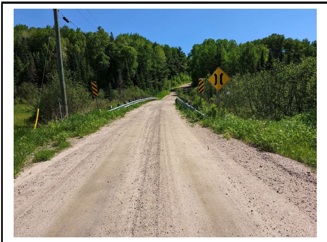
Photo 2 Structure from west approach
