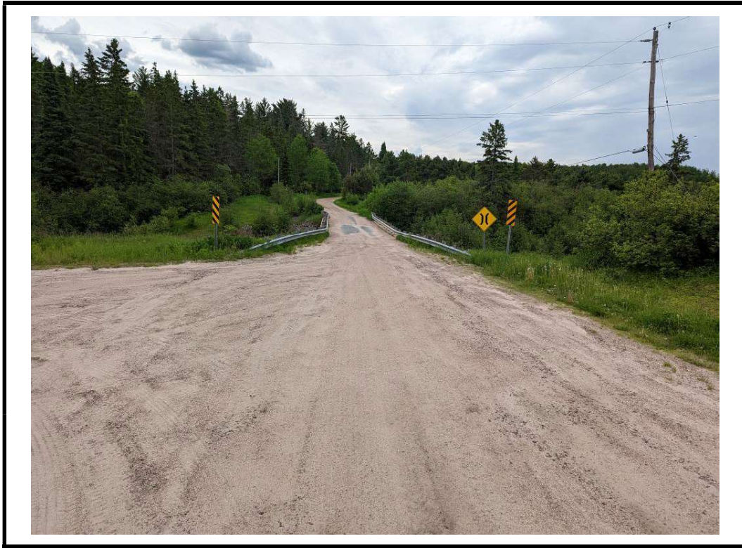
Photo 1 Structure from north approach
