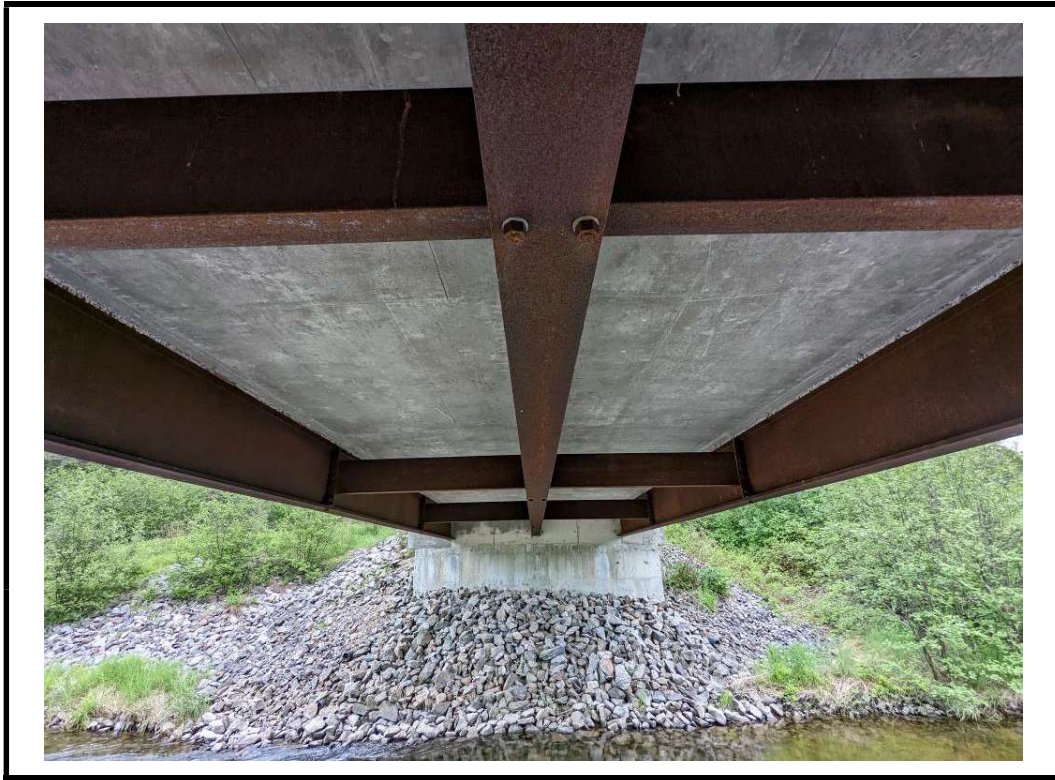
Photo 13 North underside of structure
