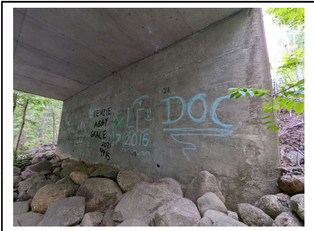
Photo 12 Typical north abutment wall
