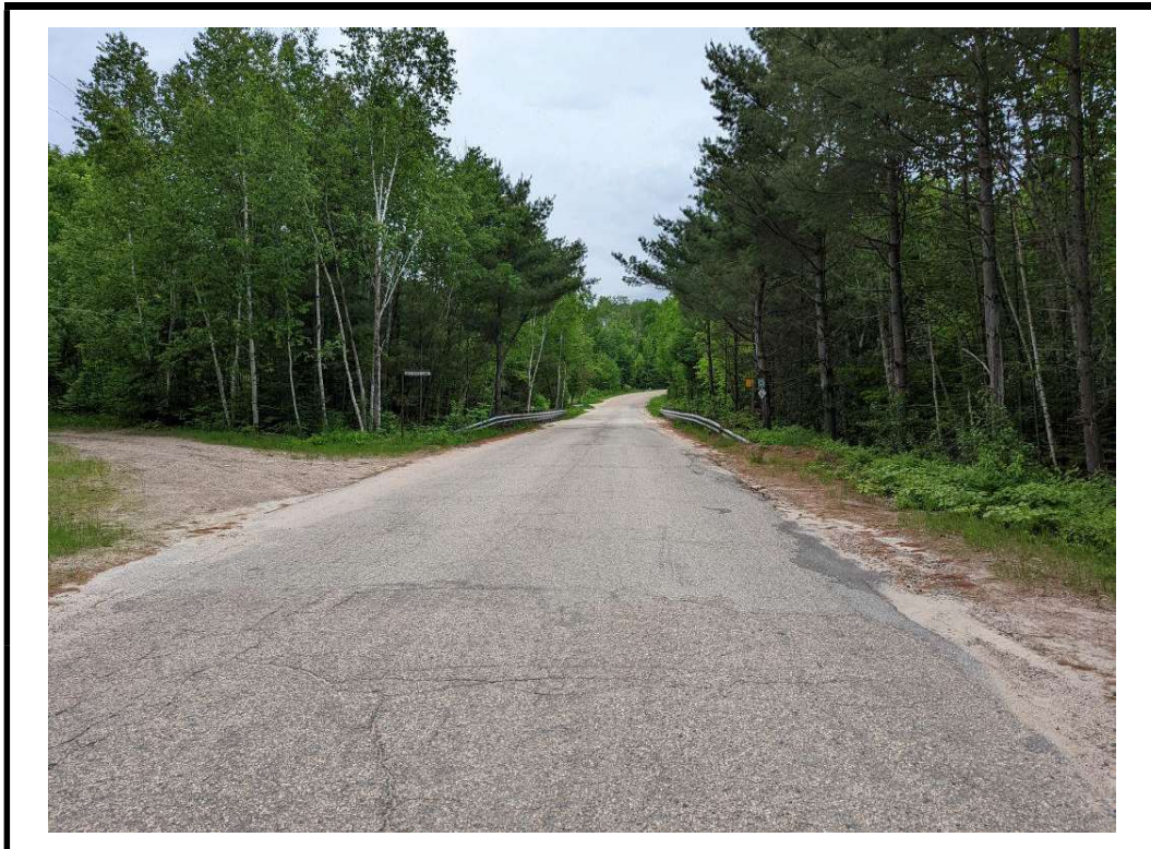
Photo 2 Structure from south approach
