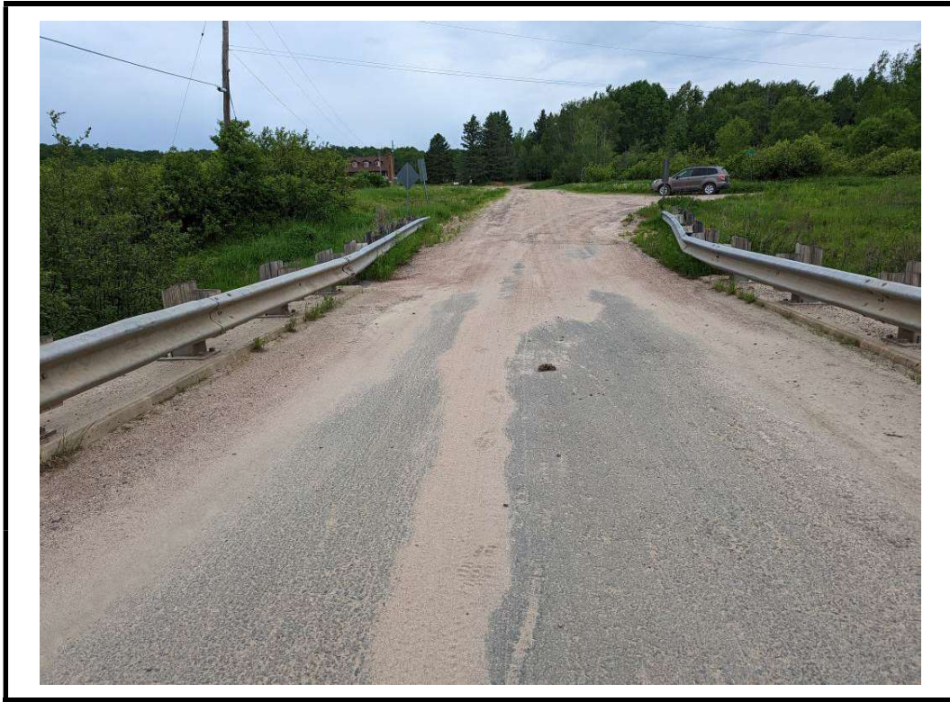
Photo 3 North approach from centre of structure
