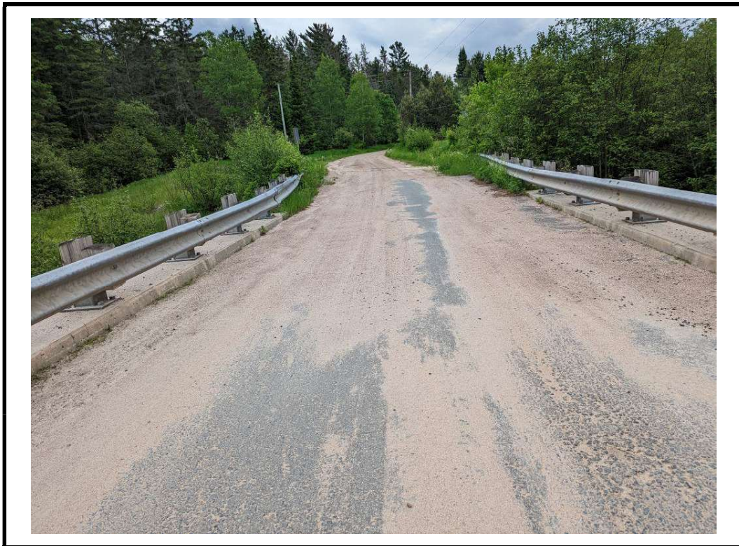
Photo 4 South approach from centre of structure
