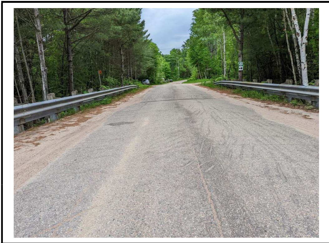
Photo 4 South approach from centre of structure
