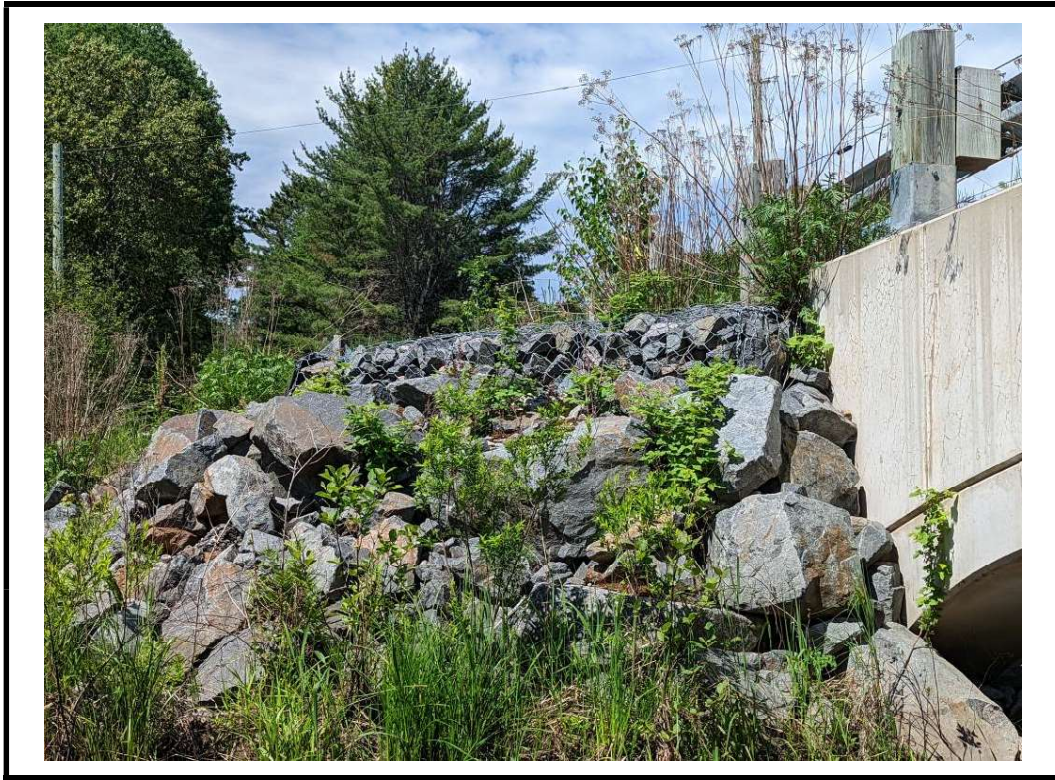
Photo 11 Typical view gabion basket wall and slope protection at southwest corner
