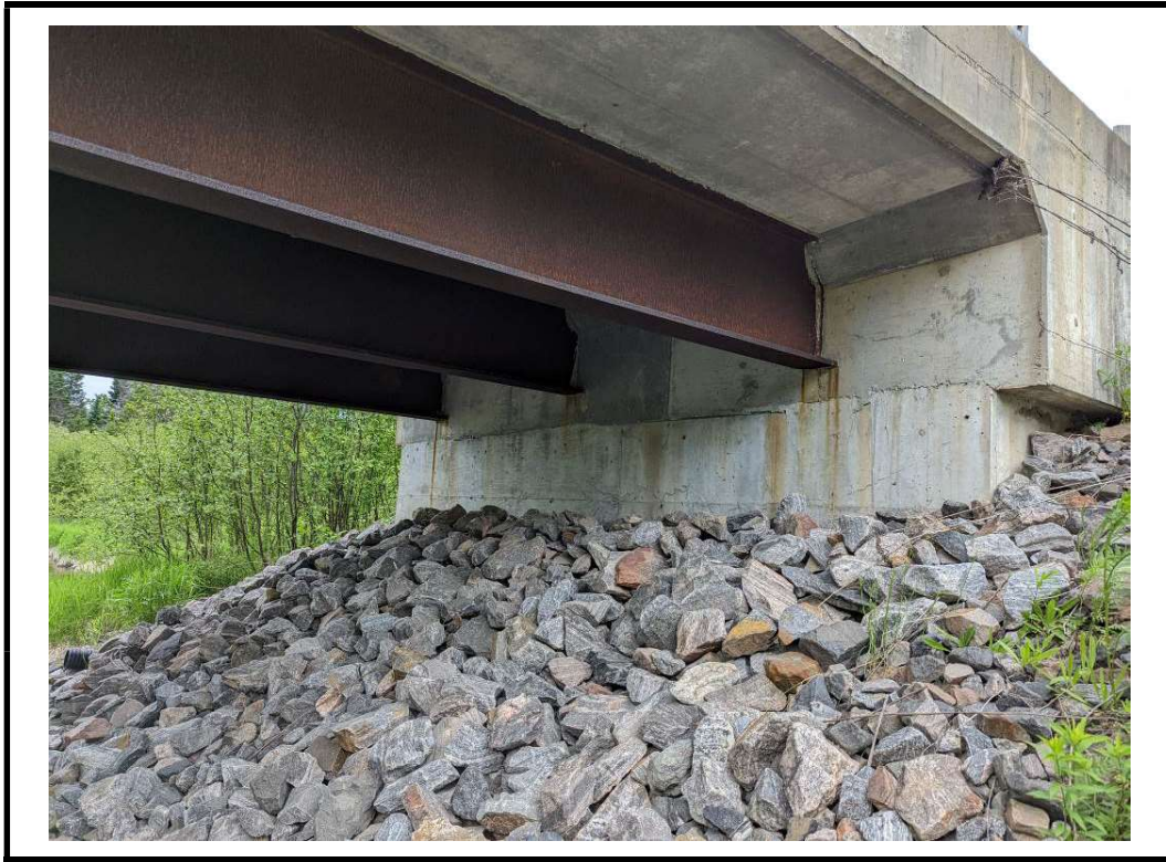
Photo 15 North abutment wall
