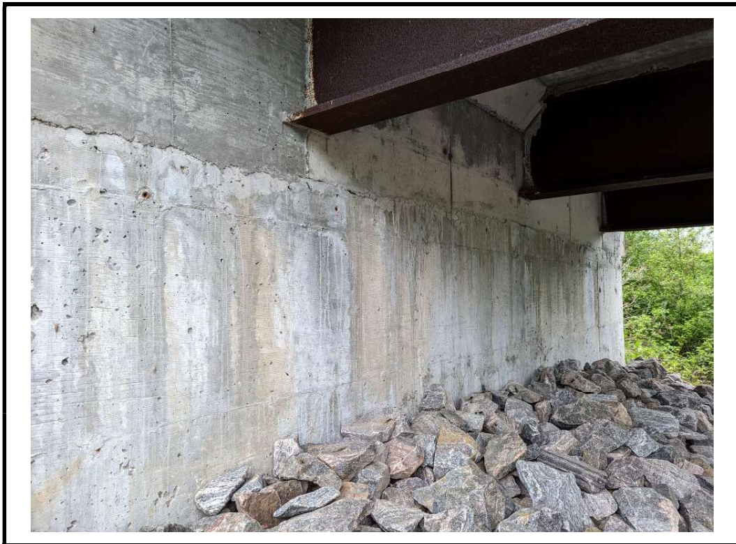
Photo 16 South abutment wall
