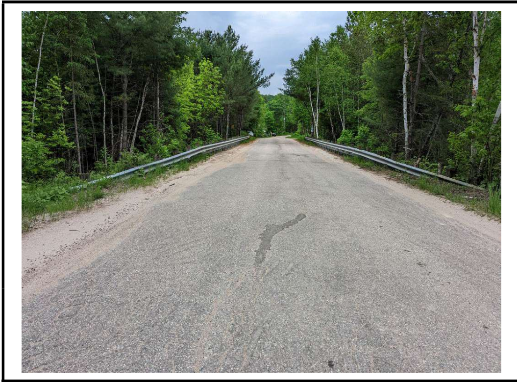
Photo 1 Structure from north approach
