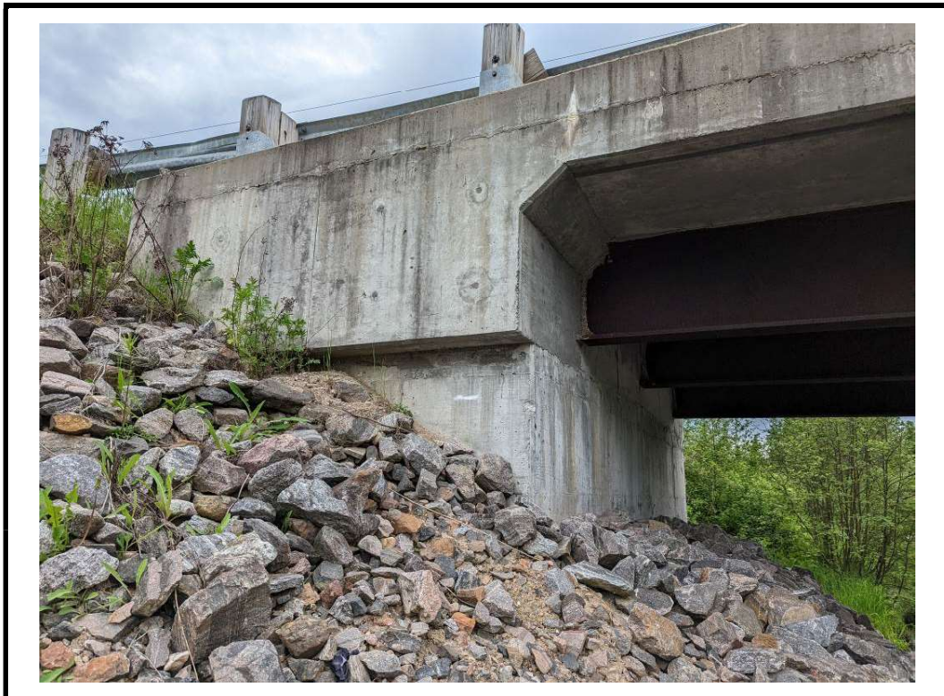
Photo 14 Typical northwest wingwall
