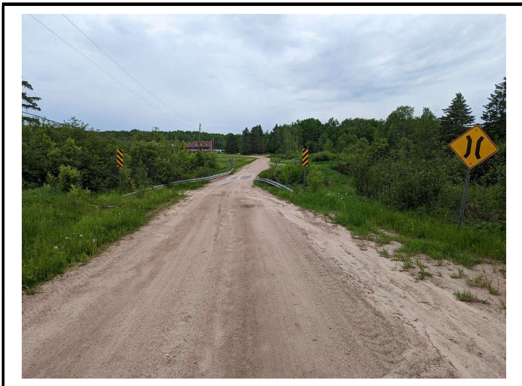
Photo 2 Structure from south approach
