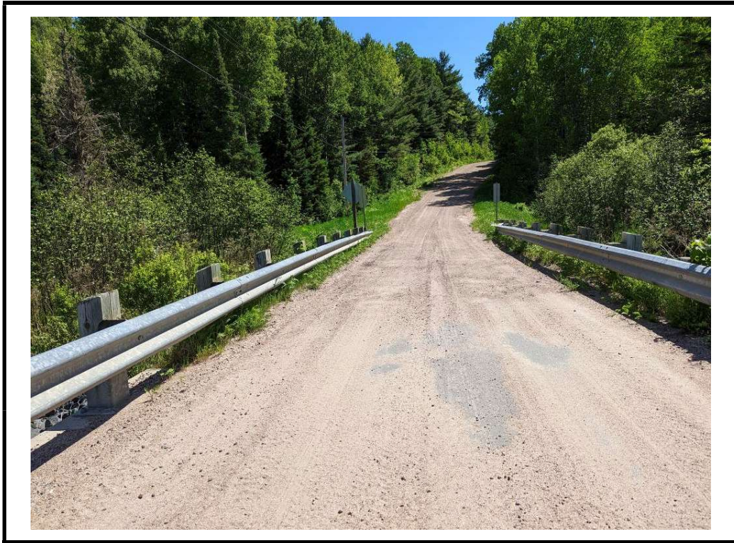
Photo 3 East approach from centre of structure
