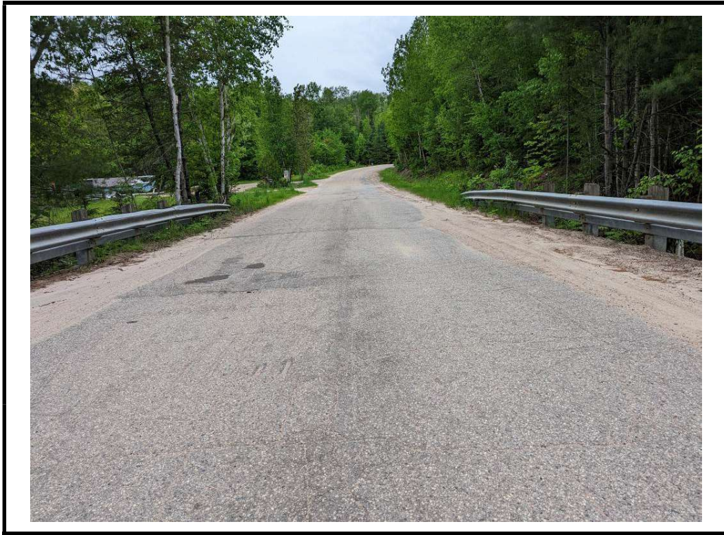
Photo 3 North approach from centre of structure
