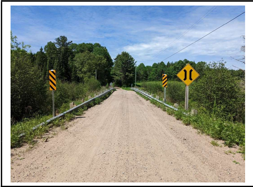
Photo 1 Structure from east approach
