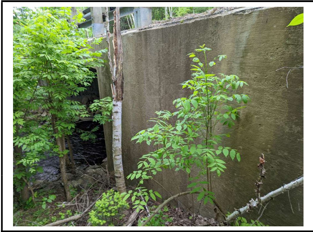
Photo 11 Typical northeast wingwall
