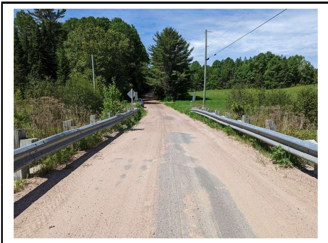
Photo 4 West approach from centre of structure
